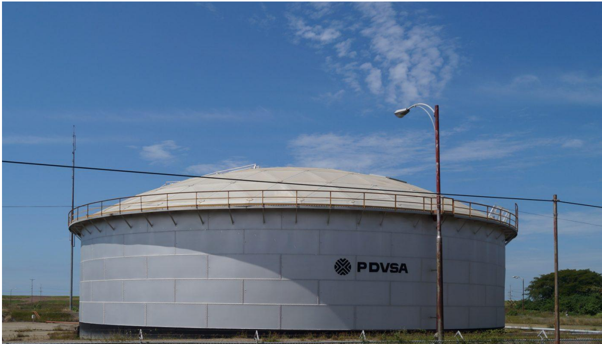
Storage tank belonging to the Venezuelan oil company PDVSA (Source: Ricastillo/Commons/CC-BY-SA 2.0 )
